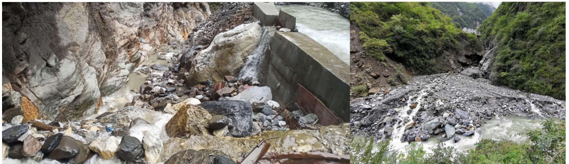
岩棚子沟取水口下游河道现状
